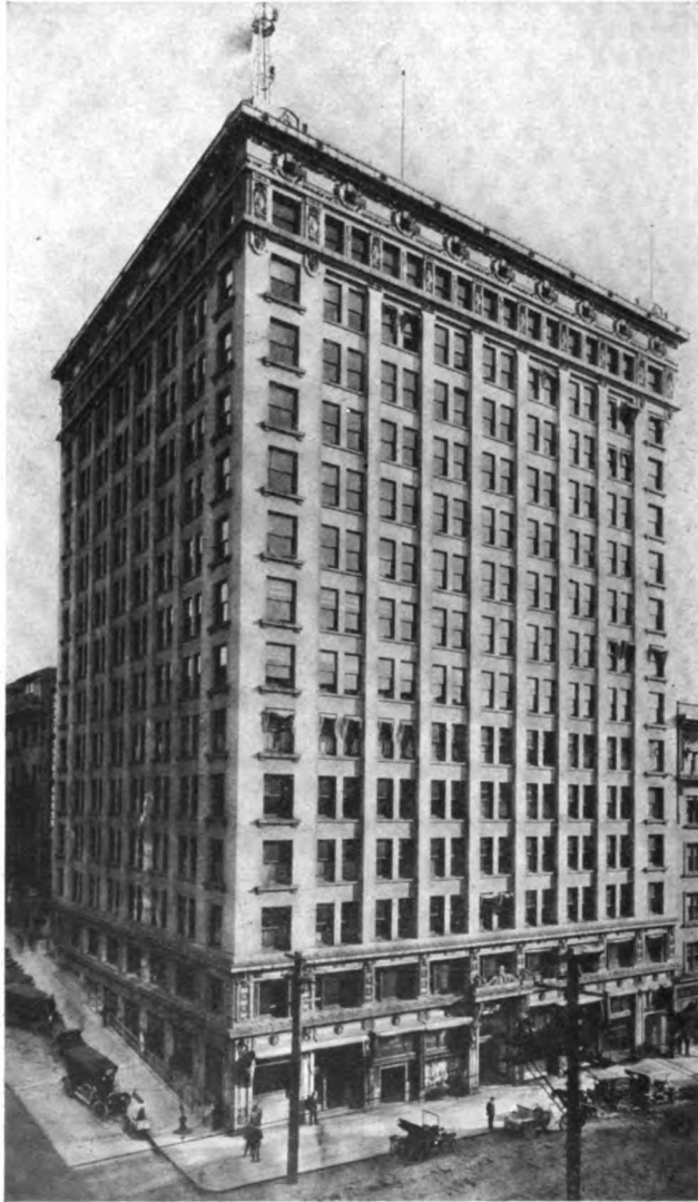
The Alaska Building—Home of the Scandinavian-American Bank.
